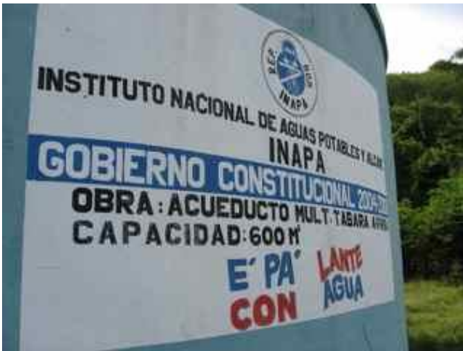
INAPA's large water storage tank north of Los Toros. This tank serves a number of other villages in the area. Capacity is 600 m 3 .
