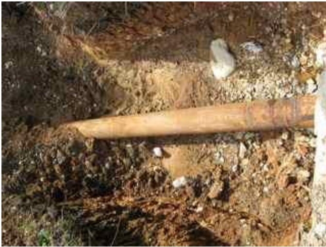
Ductile iron pipe leading from tank to Los Toros. Notice the part that was recently welded on the right side of the picture. Photo is from January 2008.
