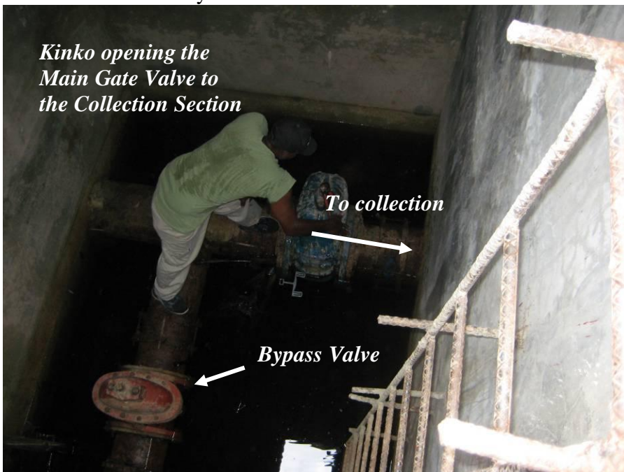
Figure 3-03: Valve Access Tank
