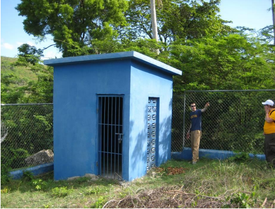
Figure 3-07: Chlorine Caseta #1 (out of service)
